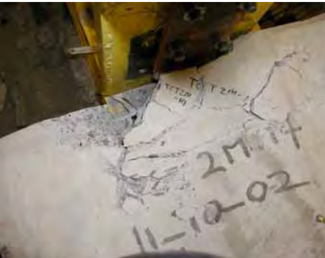
Fig. (12c). Concrete slab damage sustained as a result of testing Connector D in vertical reversed cyclic shear.
