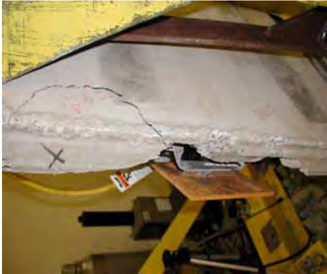
Fig. (12a). Concrete slab damage sustained as a result of testing Connector B in horizontal reversed cyclic shear.
