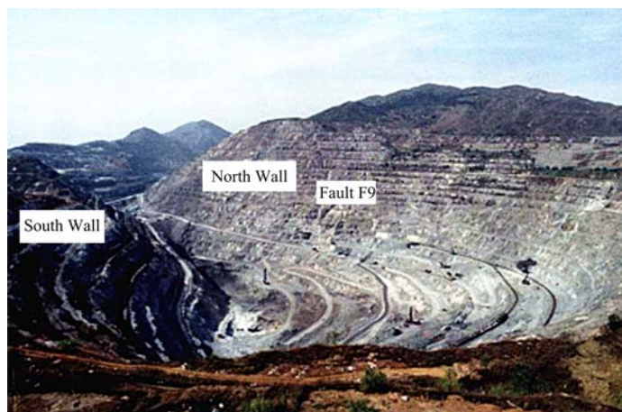
Fig. (2). The aerial photo of Daye Iron Mine and the open-pit slope.
