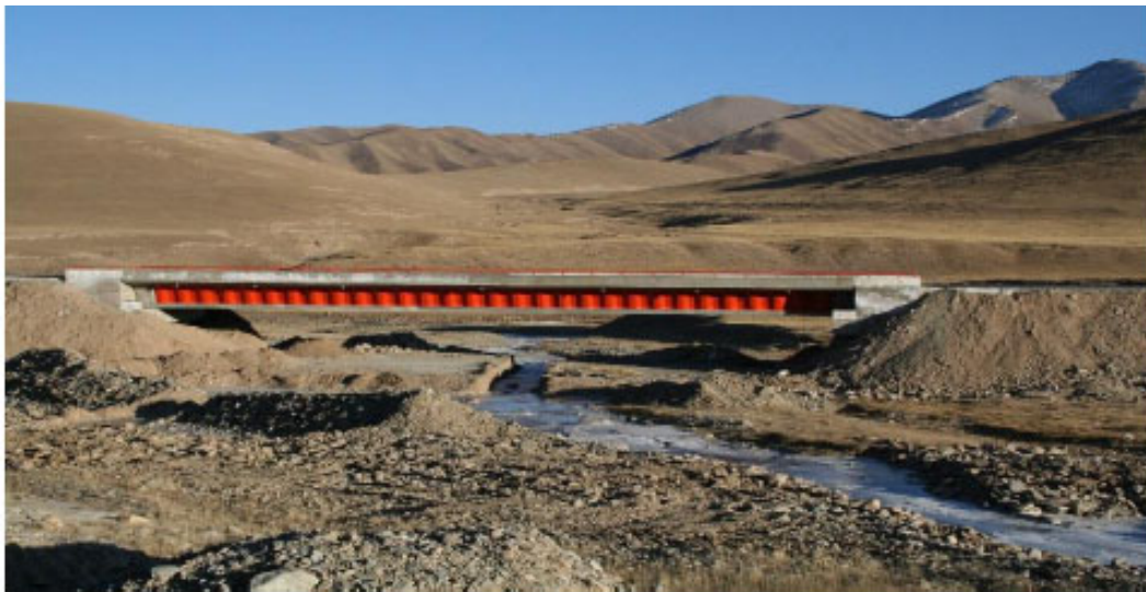
Fig. (4). Photograph of San Dao-he Bridge.
