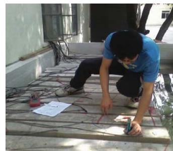
(b) Check of corrosion state
