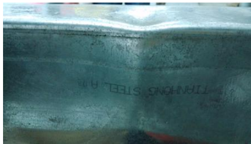
(a) Local buckling of compressive flange and web
