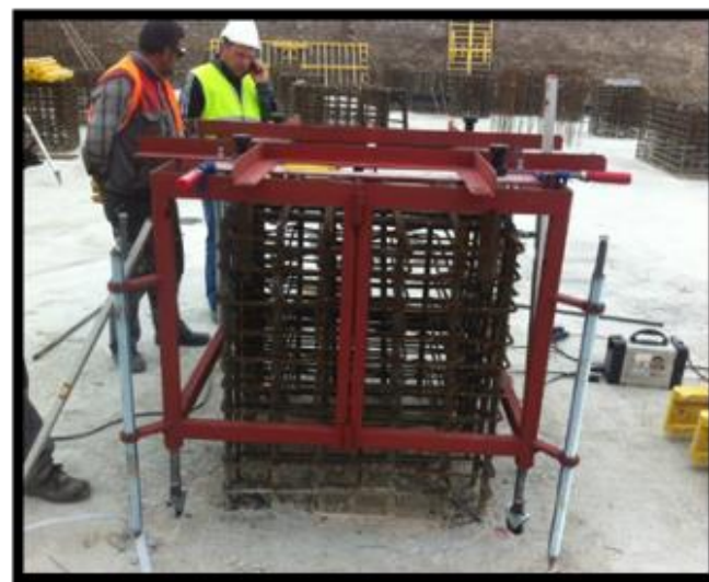
Fig. (11). Installation of bottom dowels and steel assistant table.
