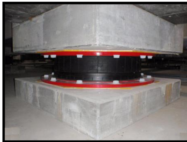
Fig. (3). Application of isolator directly to concrete.
