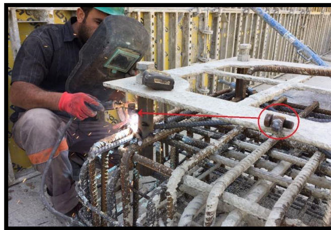
Fig. (12). Welding bolts to isolator's bottom dowels.
