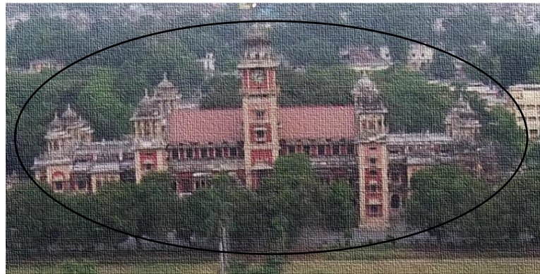
Fig. (1). 3D view of 103-year-old senate hall building, Allahabad University (Indo-Saracenic Style).
