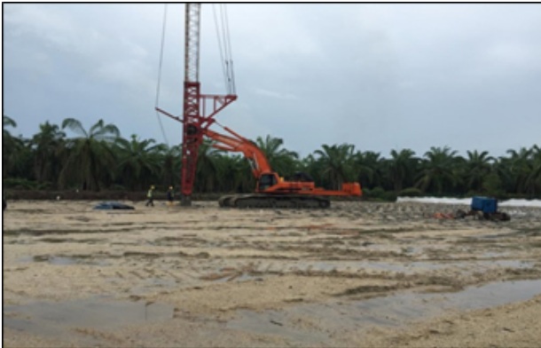
Fig. (12). PVD Installation.
