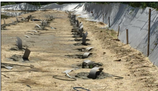
Fig. (13). Completed PVD installation according to the spacing, pattern and depth.
