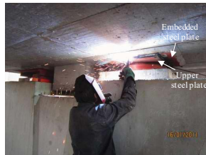
c) Welding upper steel plate with an embedded plate.
