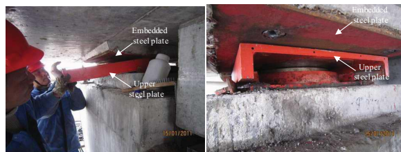
b) Replacement of upper steel plates.
