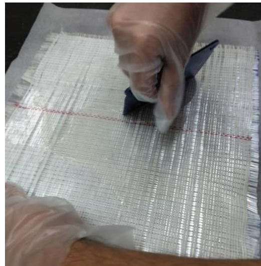
Fig. (3). Spreading the epoxy evenly on the GFRP sheet.
