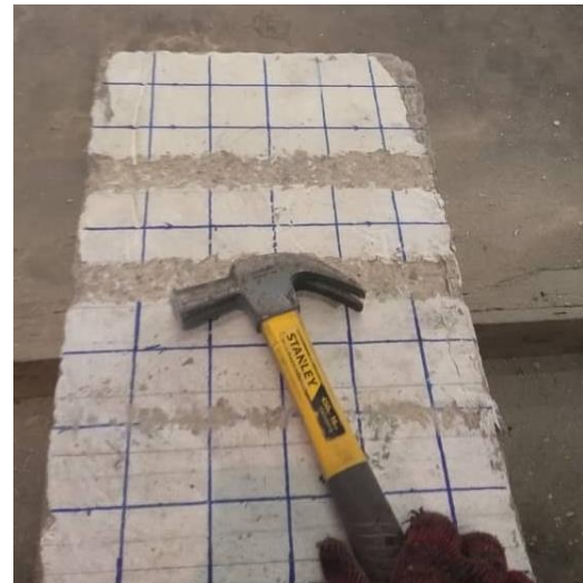
Fig. (8b). The RC beam's surface was roughened.
