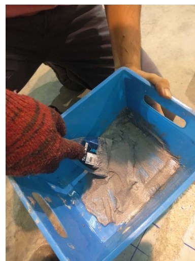
Fig. (8c). The Sikadur-30 was mixed until turned into grey color mixture.
