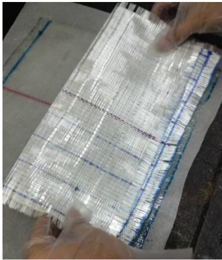
Fig. (5). Another GFRP sheet was covered on the wet GFRP and rolled again.
