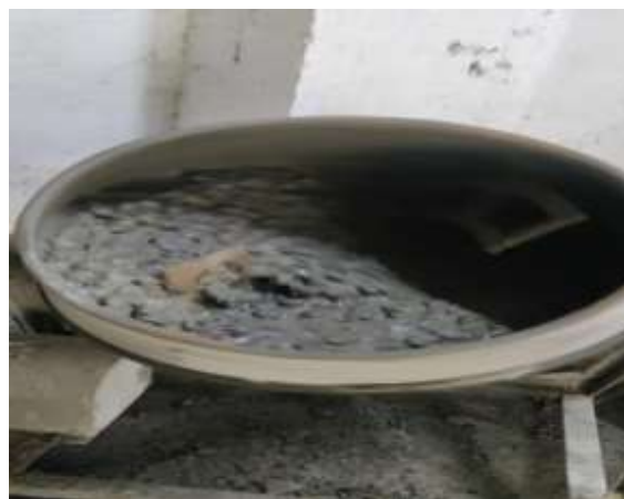
Fig. (5). Concrete mixing.
