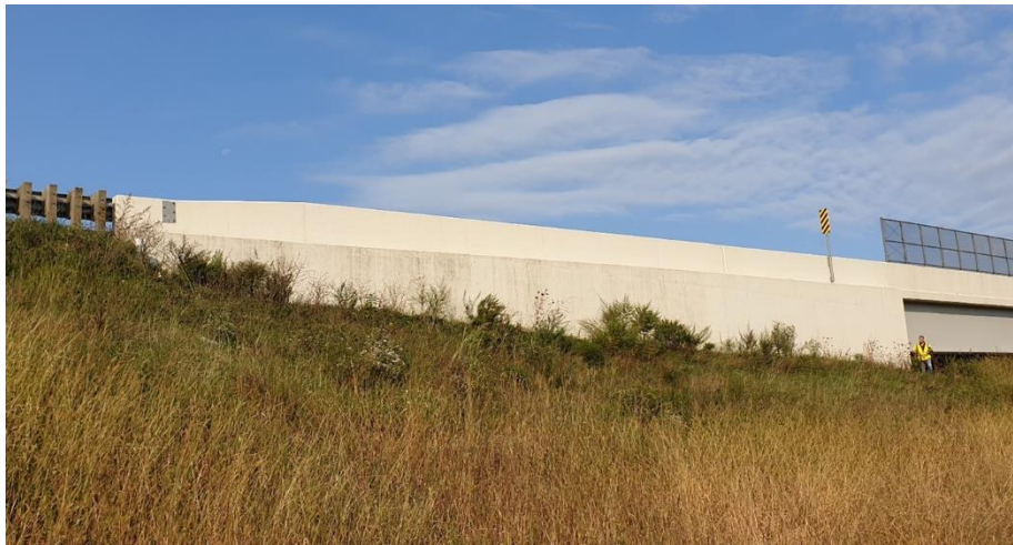
Fig. (2). CUY-77-14.35. The right forward abutment wing wall (wall 3).
