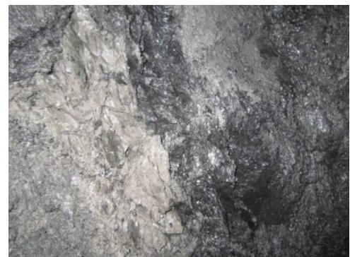
(b) Coal stratum revealed by the tunnel excavation
