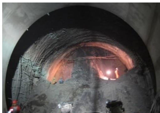
(a) Tunnel excavated in the coal stratum
