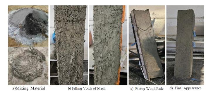
Fig. (13). Process of retrofitting using eco-friendly mortar.
