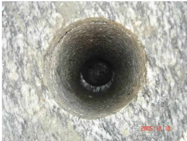
Fig. (5). Bored internal dislocation.
