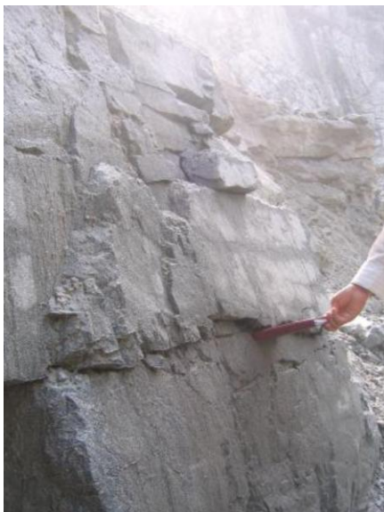
Fig. (6). Steep rock wall dislocation.
