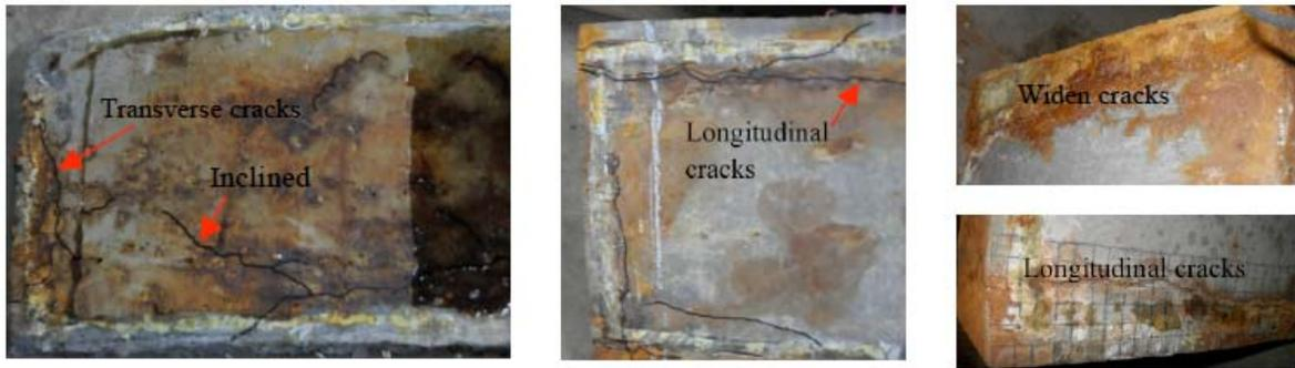
Fig. (7). Damage morphology photo of corroded segment surface.
