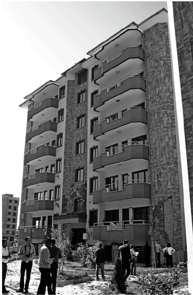
Fig. (1). Main façade of building B.
