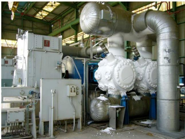
Fig. (2). Horizontal type BOG compressor.
