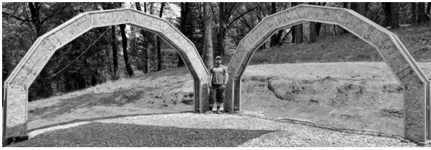
Fig. (18). First two assembled arches for a cross vault masonry frame.
