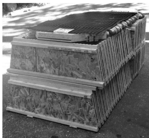
Fig. (17). Constructed block materials for a cross vault masonry frame.
