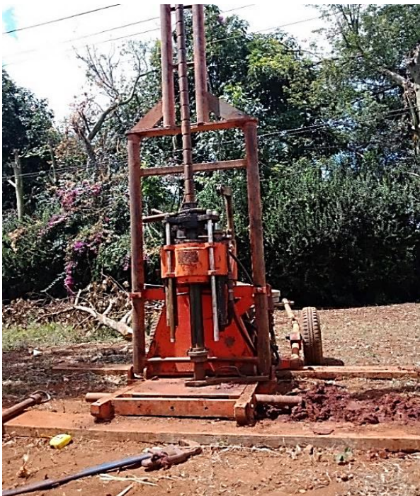
Fig. (4). Apparatus used during geotechnical drilling.
