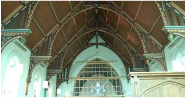
Fig. (3). Roof structure.
