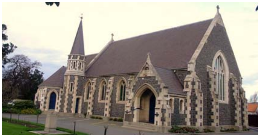
Fig. (1). General view of St. James Church.
