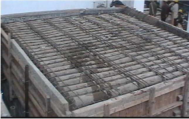
Fig. (1). Stiffening-ribbed-pipe girderless floor.
