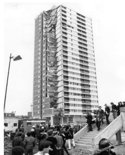
Fig. (1). The progressive collapse of Ronan Point Apartment [2].
