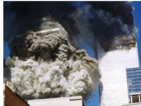
Fig. (3). The progressive collapse of WTC towers [4].
