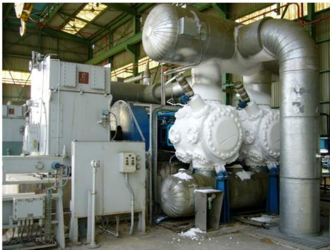
Fig. (2). Horizontal type BOG compressor.
