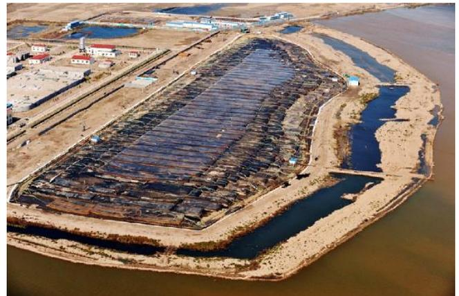
Fig. (1). The geotube dams in coastal reclamation projects.
