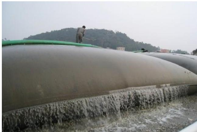
Fig. (2). Sludge dewatering by the geotube.
