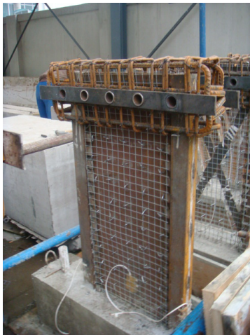
Fig. (1). Construction photograph of specimen GBW2.
